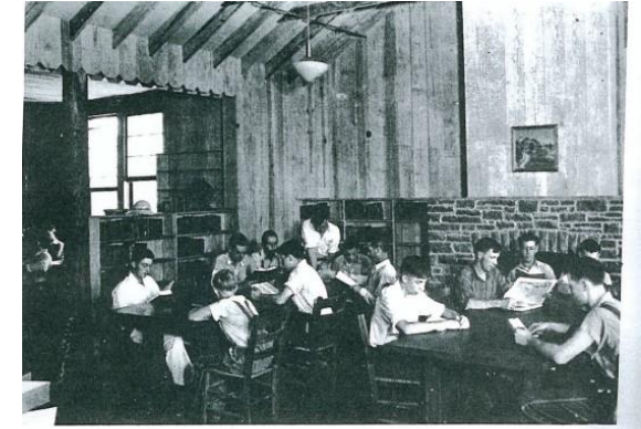
NORRIS LIBRARY—This photo, taken in 1934, shows the TVA library in Norris. Two libraries were actually established in the community, one for the school and one for construction workers who were working on Norris Dam. Mary U. Rothrock, TVA library specialist from Knoxville, had a great deal to do with the county getting its first full-time librarian.
